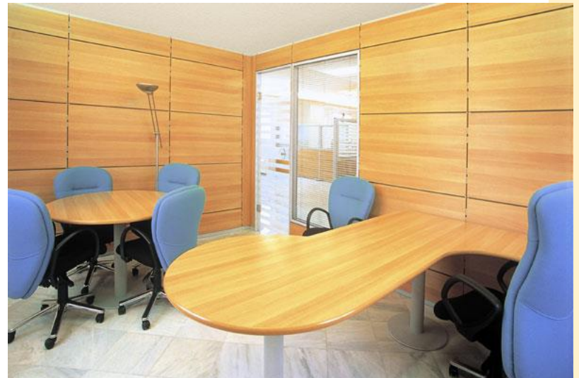
Removable partitions in a German office building
