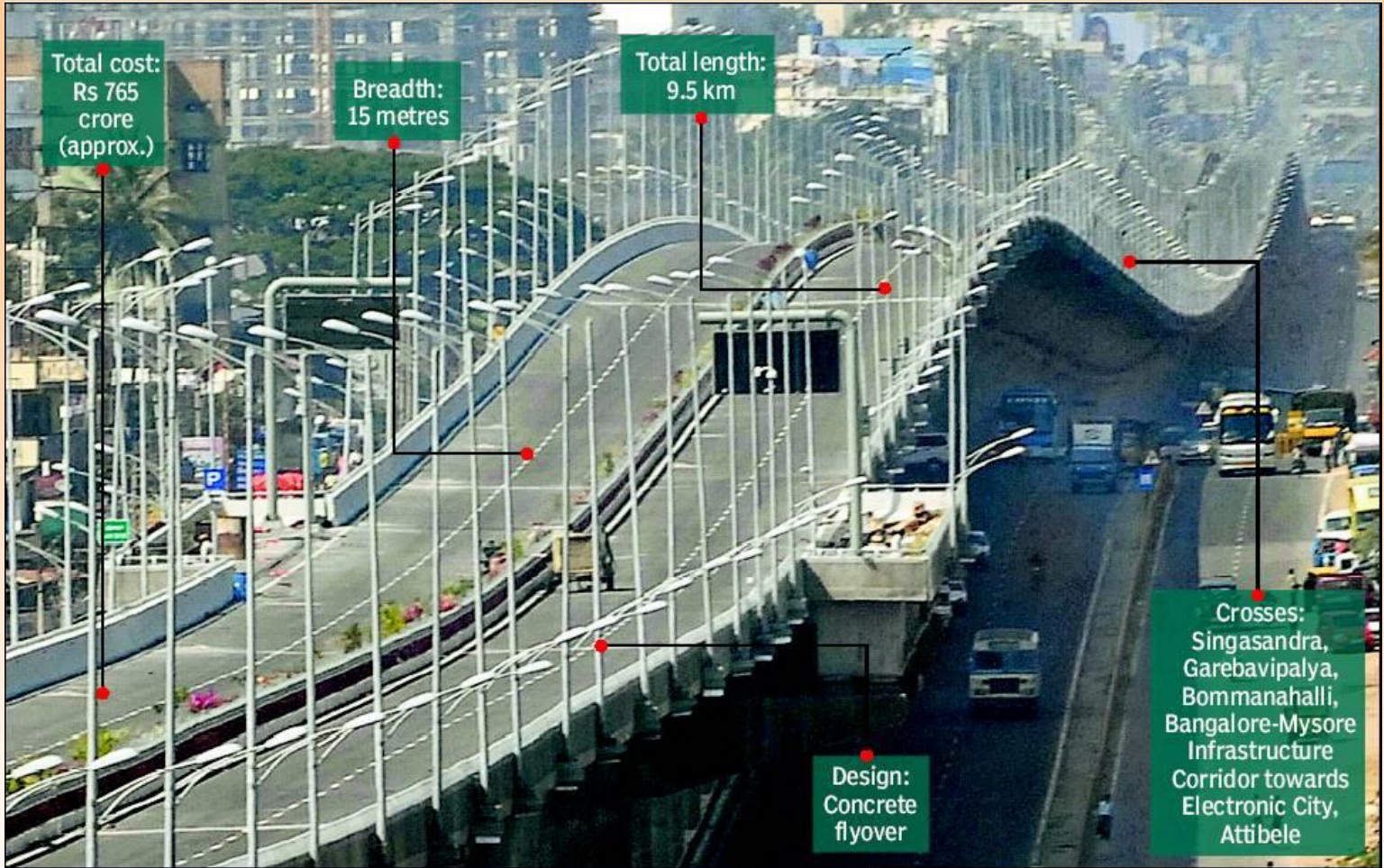
Elevated highway to Electronics City
