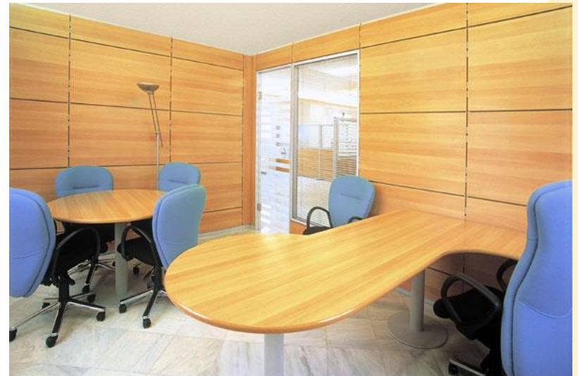
Removable partitions in a German office building
