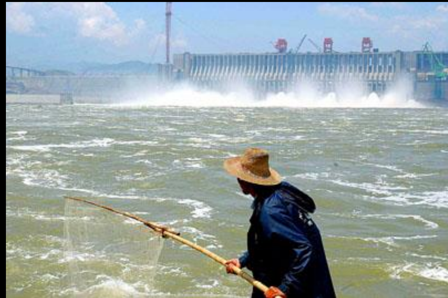
Three Gorges Dam on Yantze River World's largest hydropower dam
