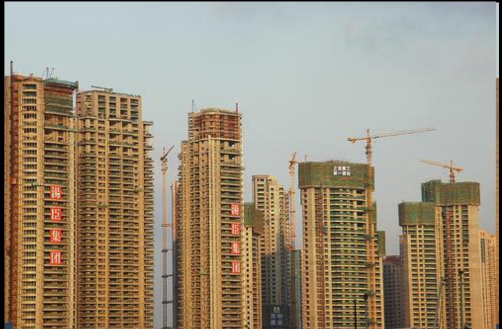
Apartment blocks under construction Shanghai
